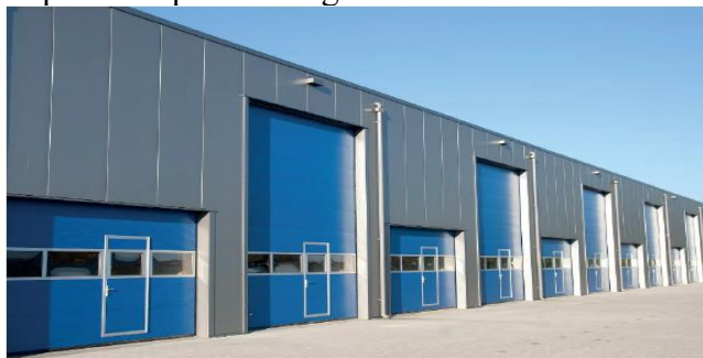
Figure 2. An industrial building constructed
