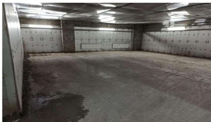
Figure 5- Humidity treatment chamber.
